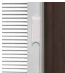
Blind operator as viewed from the interior of the home
